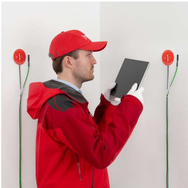
Figure 3 HFPO1 heat flux sensor and thermocouples mounted on a wall and measured with the TRSYS20 measuring system.
