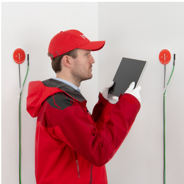
Figure 2 HFP01 heat flux sensor and thermocouples mounted on a wall.
