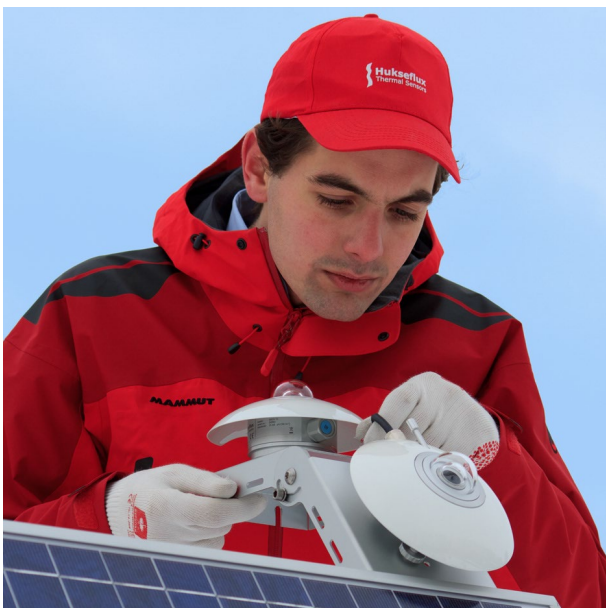
Figure 2 Dual setup in PV system performance monitoring.
